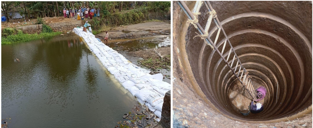
Figure 5: Water conservation works done under AUEGS in Wadakkanchery. Bund creation (left) and well construction (right) (Photos shared by the official in Wadakkanchery (left) and taken by the author (right), February 10, 2023)
