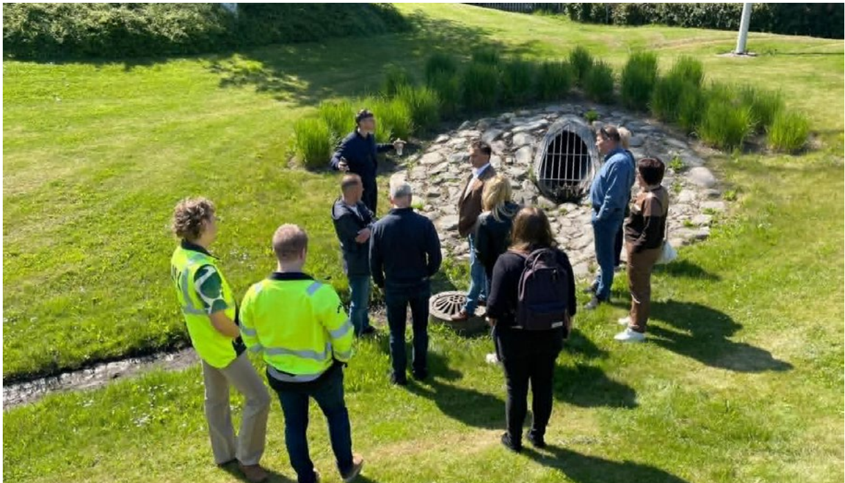
Study visit at waste water infrastructure of Ternopil in Ronneby. Photo: Ronneby kommun
